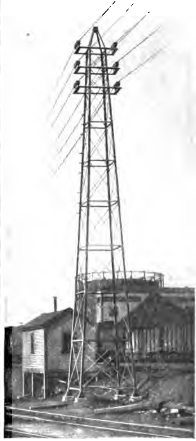
FIG. 81.—Rigid steel tower.
